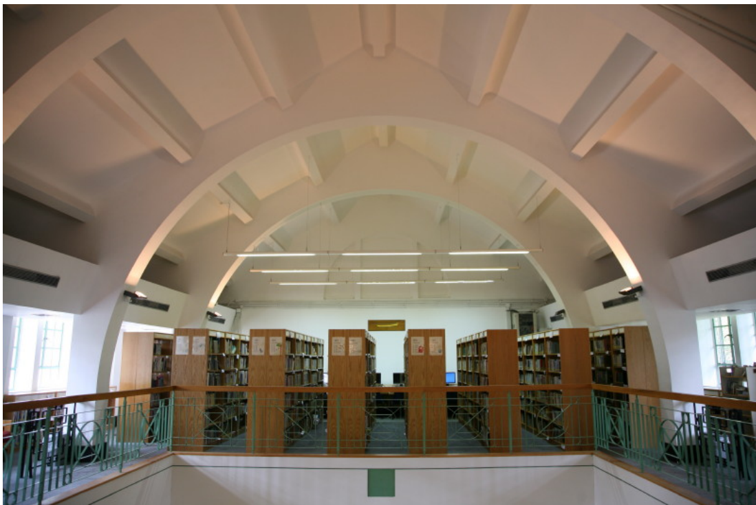
Roof of the library in the central block
