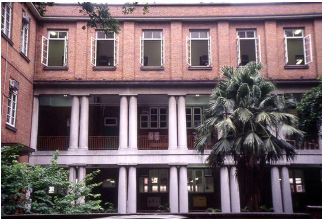
View of south wing from Bonham Road
