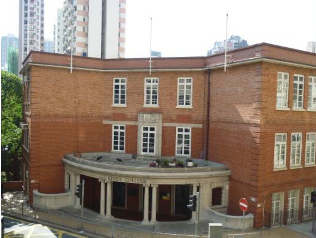
Main entrance of the school building
